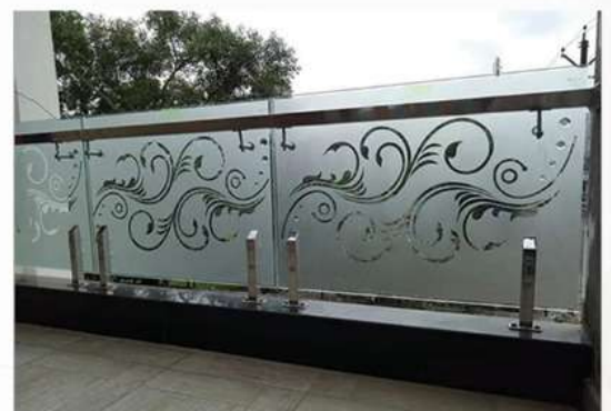
SS Glass Railing With etching
